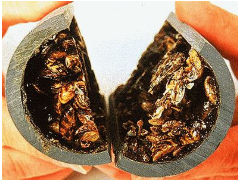
Piping Infested with Zebra Mussels
