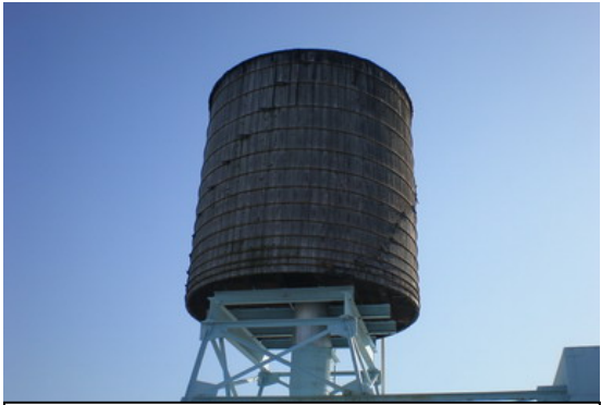
AN EXAMPLE OF A TYPICAL GRAVITY TANK
