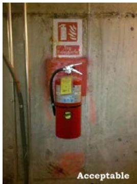
Fire extinguisher in a construction site.
