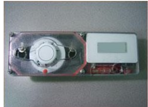
Duct smoke detectors
