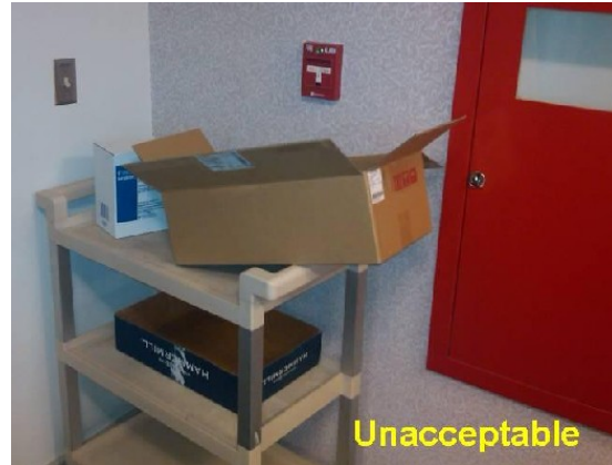
Obstructed Manual Pull Station
