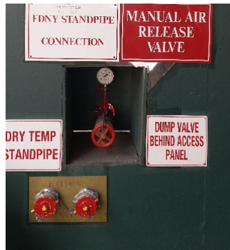
Figure 4-3. Air Pressurized Standpipe System
