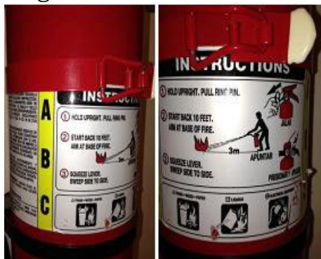
Figure 5-7. ABC Fire Extinguisher Label
