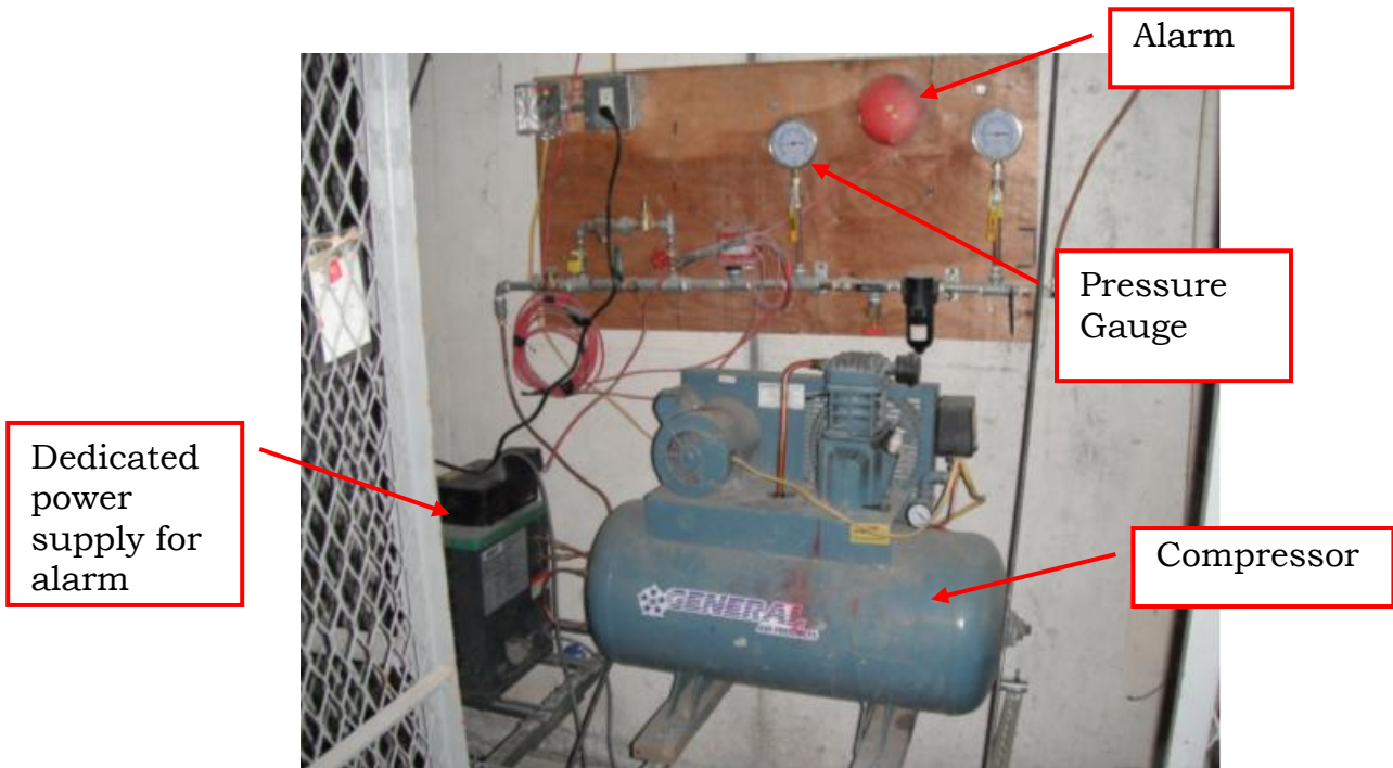
Figure 4-17. Examples of a Standpipe Compressor/Alarm Configuration
